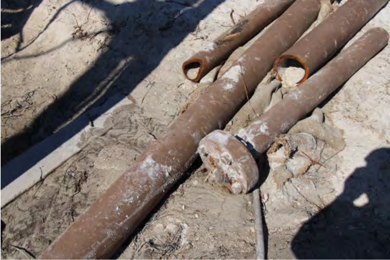
(5) The column portion broke in three places which sits at the base of the Tower waiting to be copied and reconstructed.
