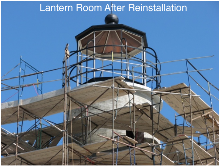
Glass Installed in Lantern Room
